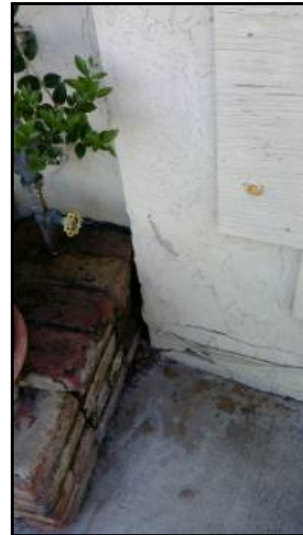
Caulk and seal all gaps, cracks and openings.
